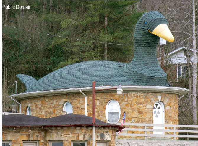
MOTHER GOOSE HOUSE, HAZARD, KENTUCKY
