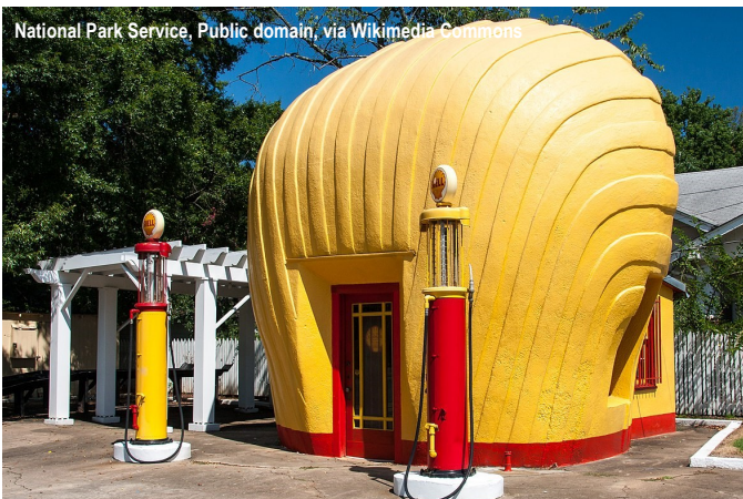
A Shell Service Station the only one to survive from eight built in the Winston-Salem, North Carolina,
