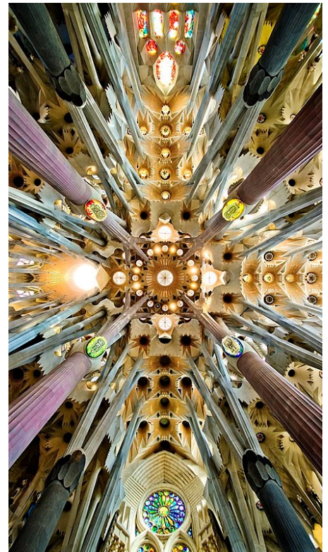
Detail looking up to the roof in the nave. Gaudí designed the columns to resemble trees and branches.
